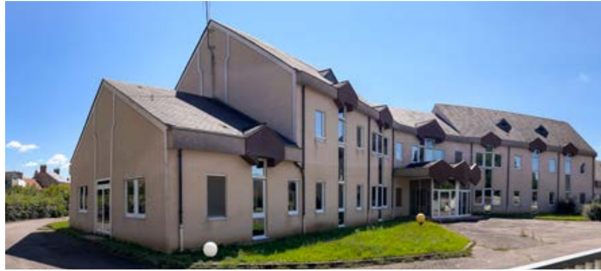
FOYER MARENGO - HABITAT INCLUSIF
